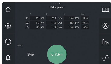
Status of reactive energy and cos fi
